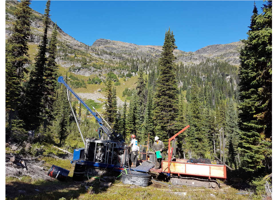
Tracked drill minimizes surface disturbance and tree-cutting
